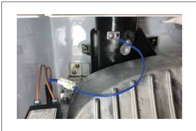
Figure 67 Exhaust Temp. Sensor
