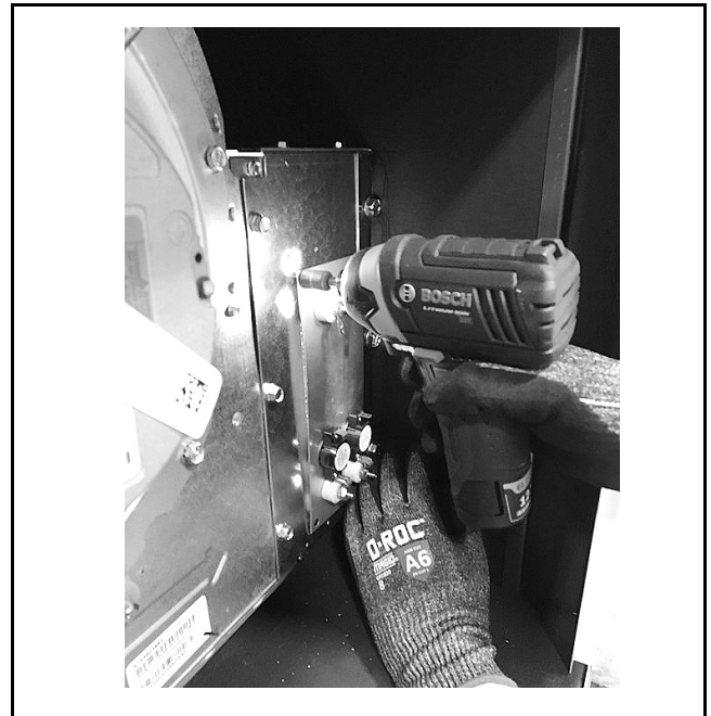
Fig. 10 Screw in the Electric Heat Element
