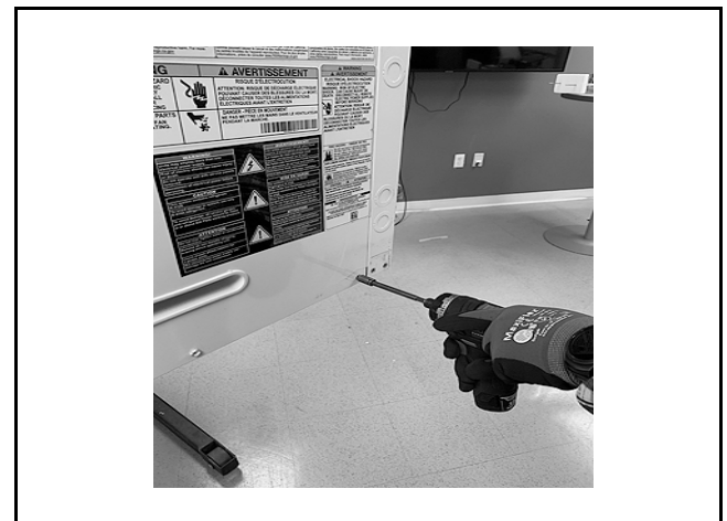
Fig. 3 Remove the Electrical Access Panel Screws
