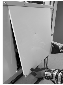
Fig. 6 Slide Out the Blower Access Panel
