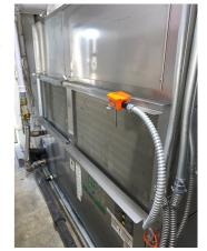
The consulting engineer and mechanical contractor particularly valued the Take-A-Part construction option. This feature allowed them to maneuver the condensing and air handler sections through the building doorways and elevator lifts separately, a requirement due to the tight spaces leading to the mechanical room.
