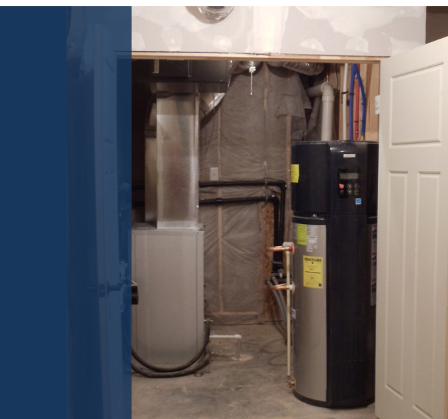
Bosch Compress heat pump water heater (right) provides DHW, and geothermal heat pump (left) provides space heating and cooling.
