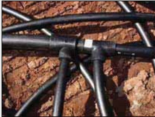
Fig. 53 Closed header Courtesy of International Ground Source Heat Pump Association/Oklahoma State University
