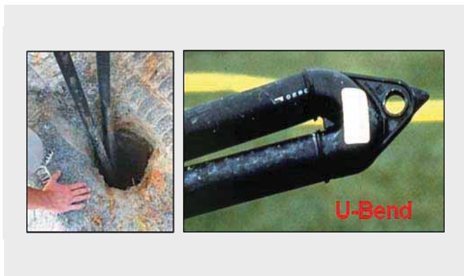
Fig. 55 Single loop with U-bend
