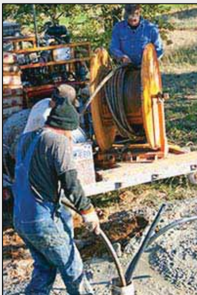
Fig. 66 Trailer mounted grout unit Courtesy of International Ground Source Heat Pump Association/Oklahoma State University
