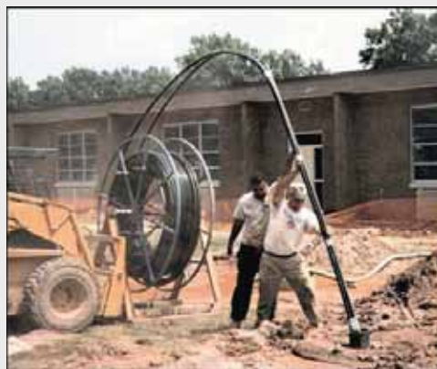
Fig. 70 Tremie / Conductor Pipe
