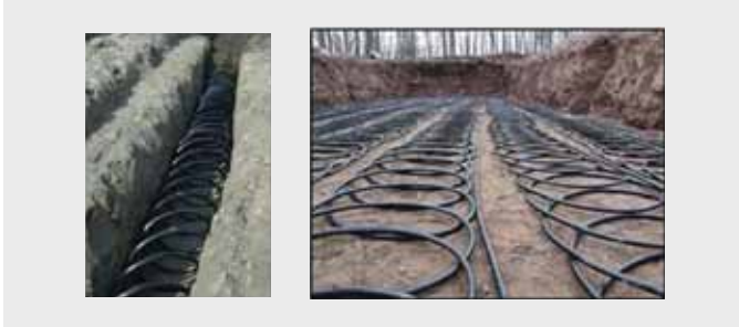
Fig. 85 “Slinky™” loop system Courtesy of International Ground Source Heat Pump Association/Oklahoma State University
