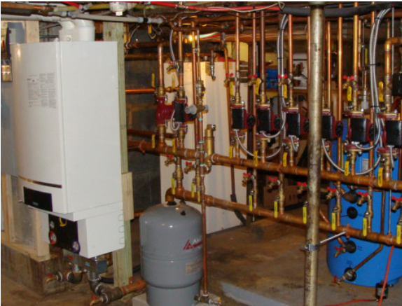
Buderus GB162 gas condensing boiler (foreground, left) and ST200 indirect water storage tank (blue, at right). Existing direct-fired water heater (white, in background) delivers high-temperature hot water to the kitchen dishwasher.
