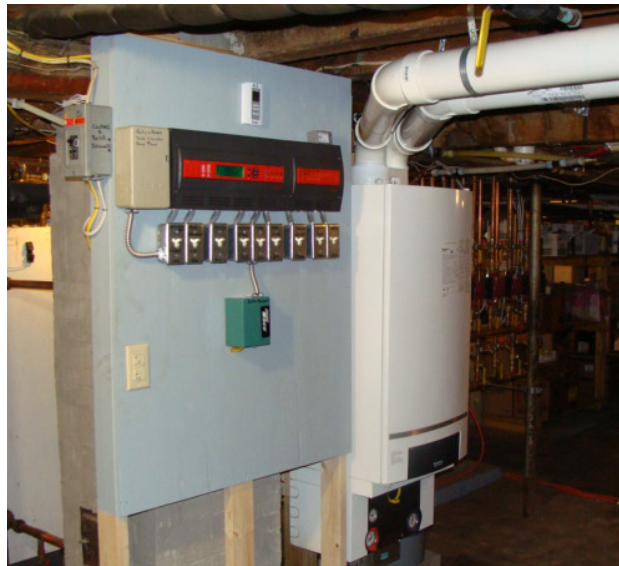
Buderus GB162 gas condensing boiler vents outdoors with PVC pipe.
