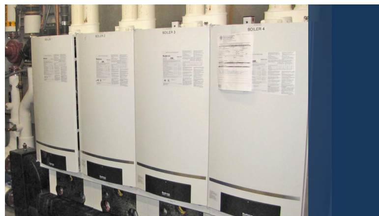
Four Buderus wall-mounted GB162 condensing gas boilers saved valuable floor space.
