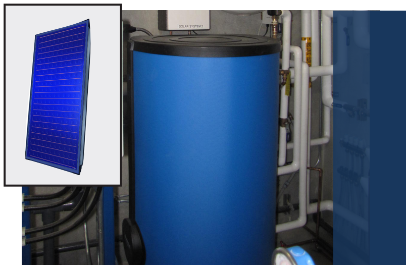
Buderus SKS solar thermal collectors (top left) provide much of the building's domestic hot water (stored in Buderus tank, center), saving significant annual energy costs.
