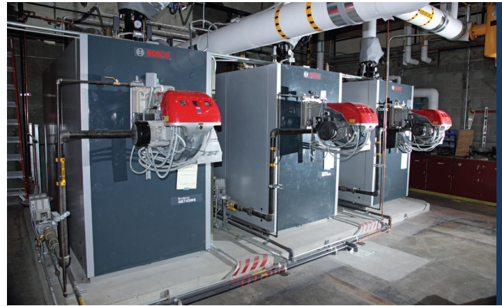
Three Buderus SB745 gas condensing boilers are installed in Redmond High School.
