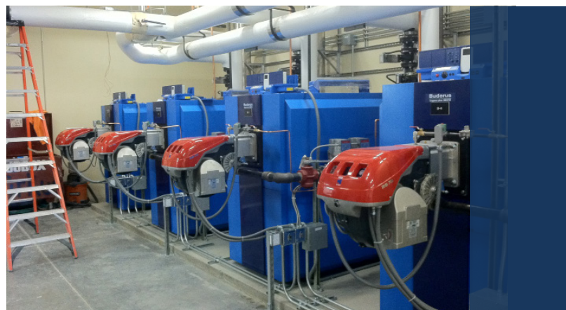
Four Buderus SB615 gas condensing boilers at Ridgeview High School
